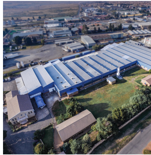
Grinding Techniques headquarters in Chamdor (Krugersdorp)
